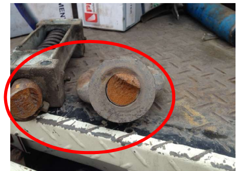
Picture 2 – The above picture shows where the ring feeder shaft has been bent through jack-knifing the trailer, causing the shaft to fail.
